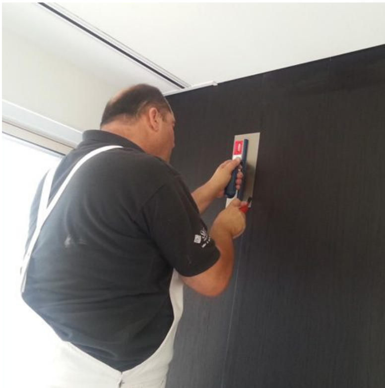
Double cutting the seams
