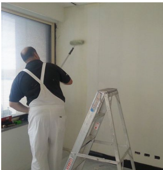
Priming the wall surface
